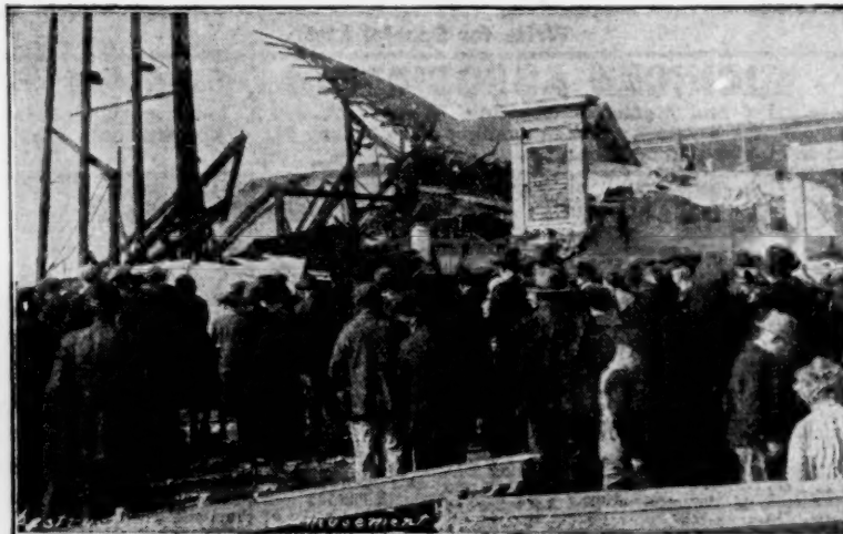
The fire which swept Venice Pier, Venice, Calif., a few weeks ago destroyed many of the amusement devices and left the greater part of the pier a mass of twisted ruins. The above photo shows a part of the ruins. The pier is now being rebuilt.
